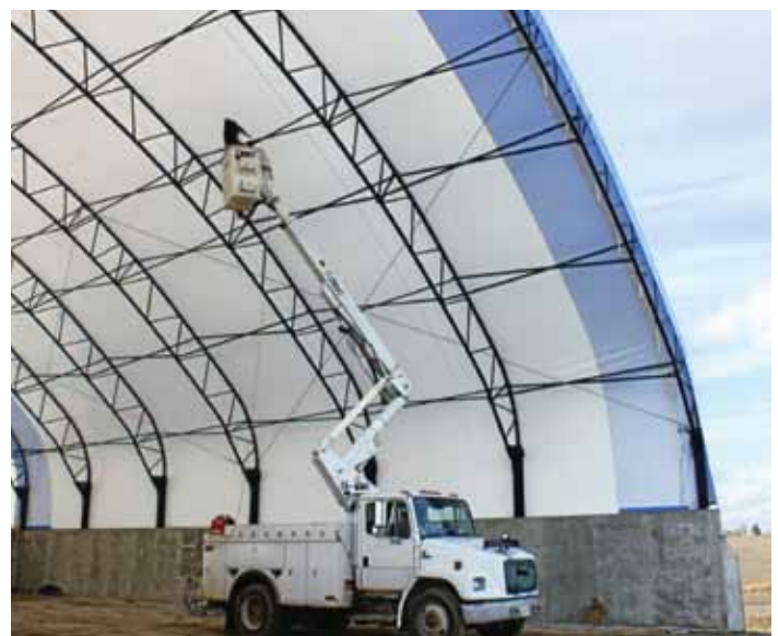
Accu-Steel repairs original structure.
