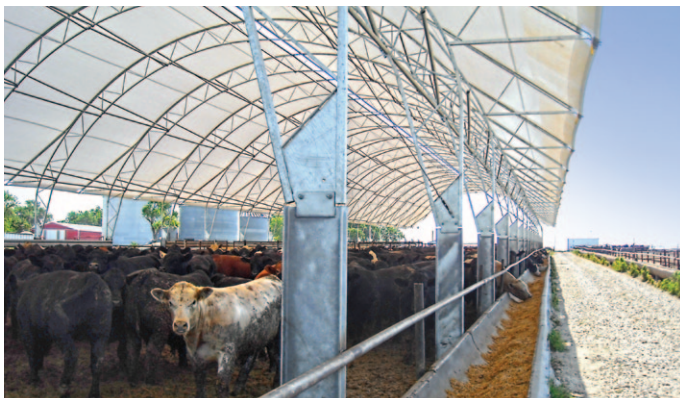
Cattle building 60 ft. by 512 ft.
