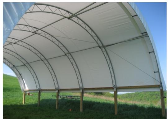
Inside Cable Installation and Bracing
